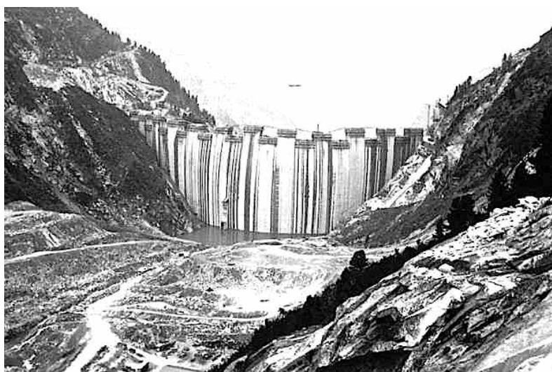
The dam for the Zillergründle reservoir under construction
